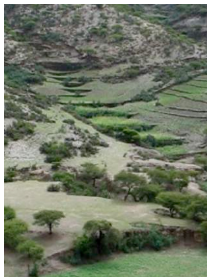
Picture 2: Check dam sequence constructed by local farmers with cultivated maize fields in Daya/Alitena,
