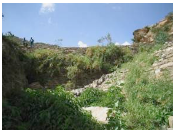
Picture 3: Topmost check dam of the Dogogola sequence, with soil stabilizing stone embankment at the right side
