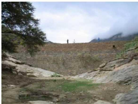
Picture 8: Front view of the Alakalo check dam; July 2003
